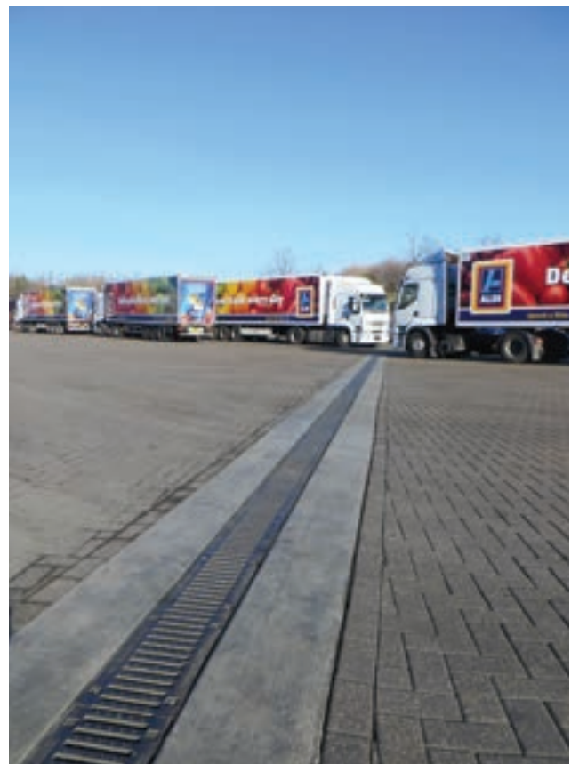
ALDI Regional Distribution Depot Darlington
