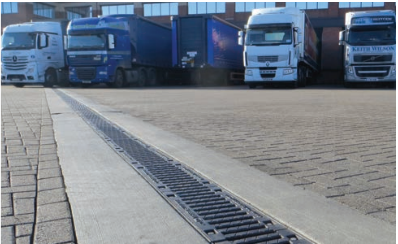
ALDI Regional Distribution Depot Darlington
