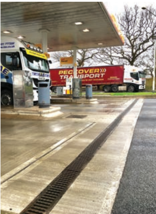
Charnock Richard Services HGV Refuelling Station
