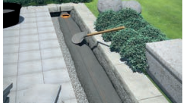
Fill with concrete and compress to foundation.
